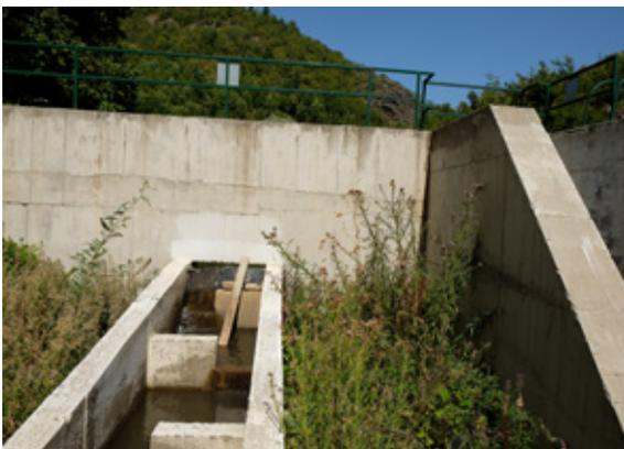
Figure 29: Blocked fish pass
