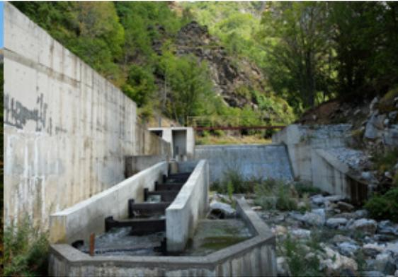
Figure 25: The intake with the new fish pass
